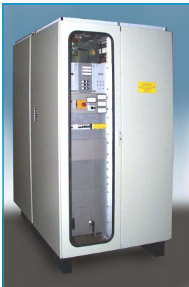
HCK 150000M - 12000 12kV / to 35 A customer specific design, 4-fouled 19" cabinet, cubical
